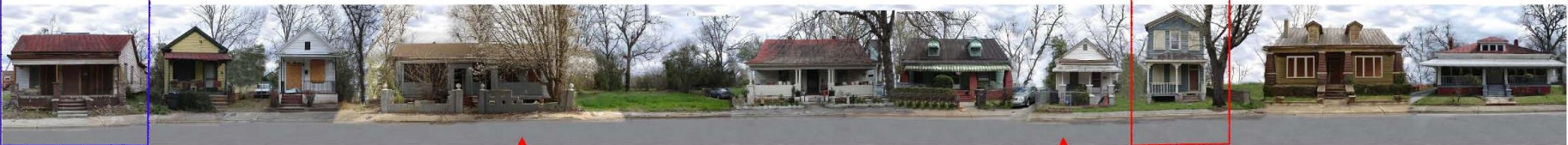
East Pine Street: Pre-construction
