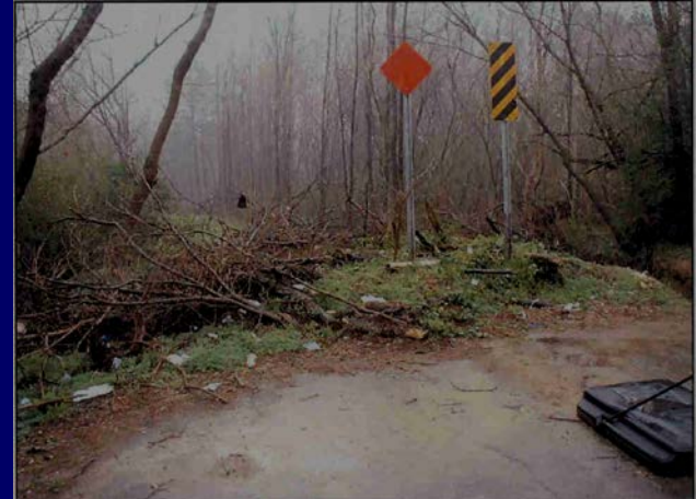
Inadequate Street Layout
